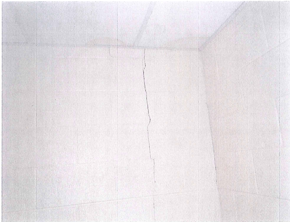
PHOTO 11 - Interior Crack At Stairs To Auditorium Stage (Near Rear Wall)
