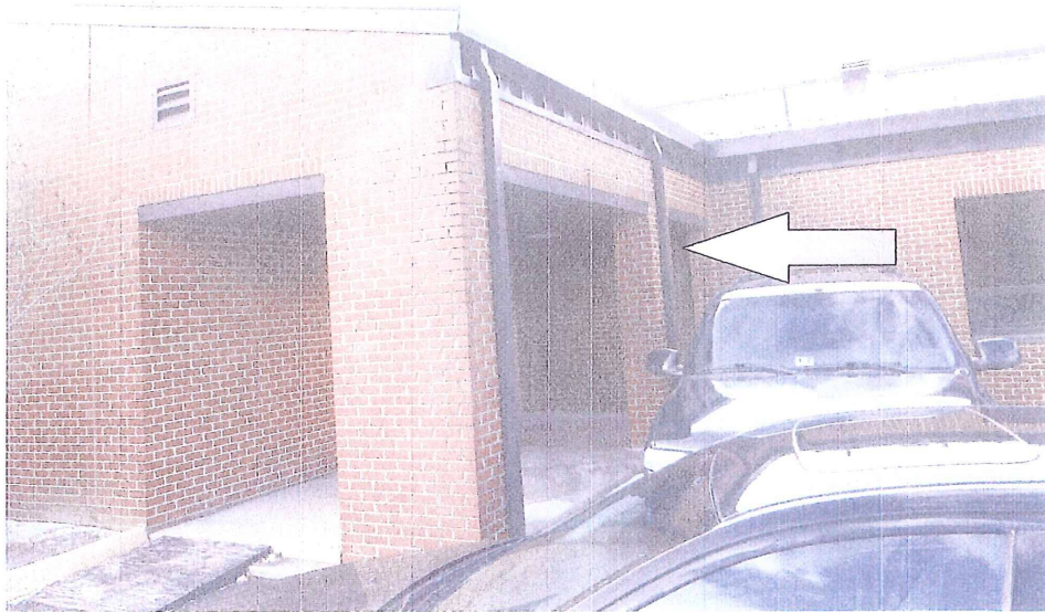
PHOTO 13 - Location of Column Shown in Photos 14m, 15 & 16
