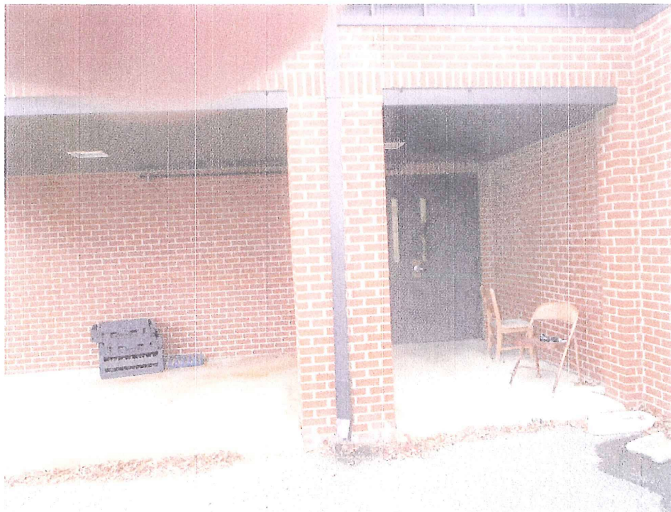
PHOTO 14 - Brick Column Shown in Photos 15 & 16
