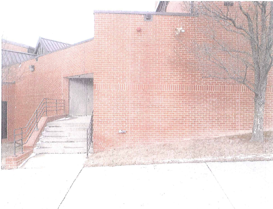
PHOTO 8 - Exterior Wall At Stairs to Auditorium Stage
