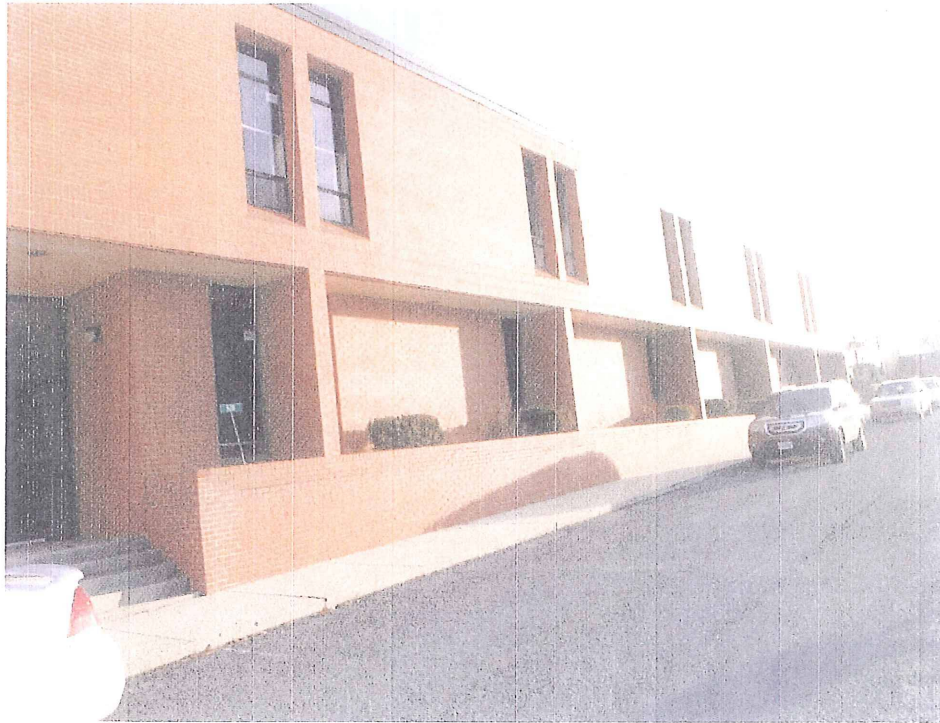
PHOTO 1 - Front of Structure ( Beam Supports Brick Just Below Windows)
